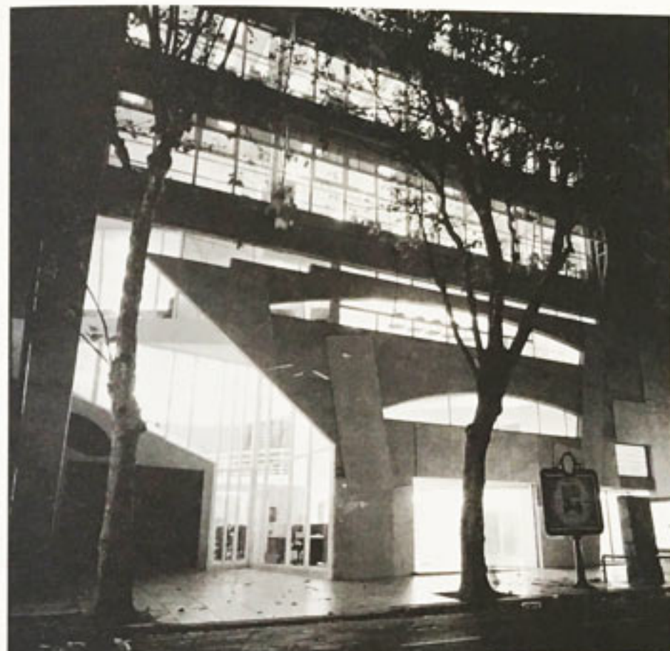
This is an extension to the existing institutional building. The new building holds the administrative offices. The floor plan is free with an only central column and concrete is the predominant element in the facade: continuous windows with sun shades of perforated steel plates, changing the image of the common office building type. Colegio de Escribanos de La Capital Federal Project: Claudio Testa, Juan Fontana, Arqs., Estudio Sevi de Arquitectura (Emel Sevi, Gerdo Sevi, Osvaldo Basso, Victor Derka, Arqs.) Capital Federal, Buenos Aires, Argentina, 1999. Photos: Diego Trolliet.
